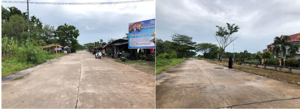
FIGURE 4. Road to STIE campus
