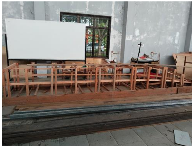
FIGURE 5.. Installation of longitudinal construction (source: activity documentation)
